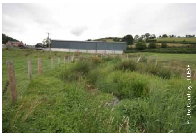
Figure 17. Fully vegetated in-ditch wetland.
