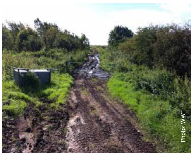
Figure 3. Runoff into farm track.
