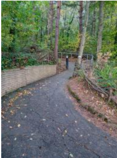
Path slope to centre from main car park
